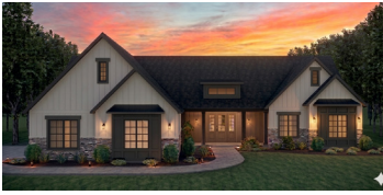
22 | MUSTON CONSTRUCTION 8785 10 MILE RD ROCKFORD 49341
